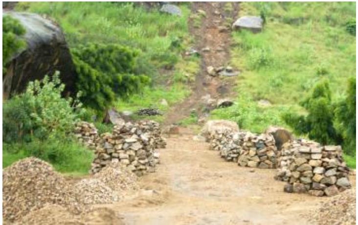
These piles of rocks were all crushed by hand. Photo by Dan Driedger
