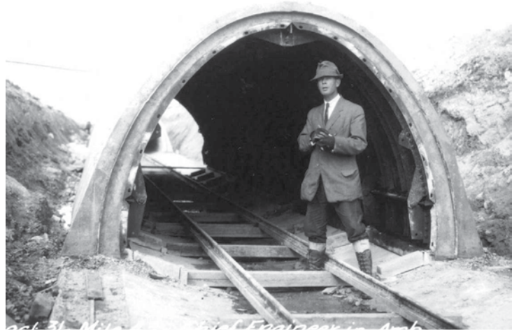
Building the Shoal Lake Aqueduct
