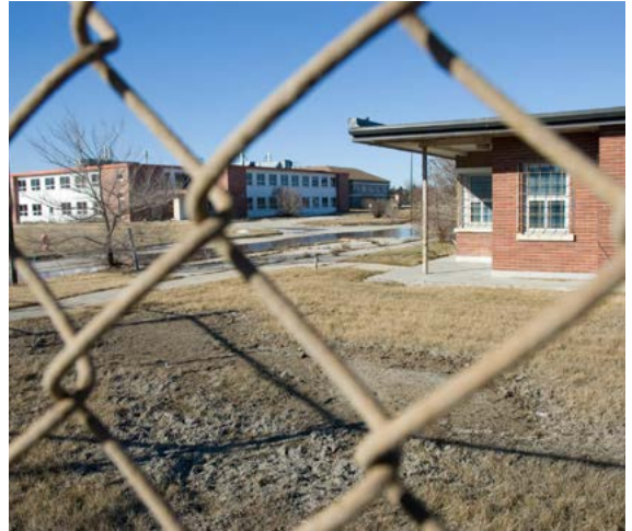
Kapyong Barracks sits empty in the heart of Winnipeg - it could become an urban reserve. PHOTO: MENNONITE CHURCH CANADA
